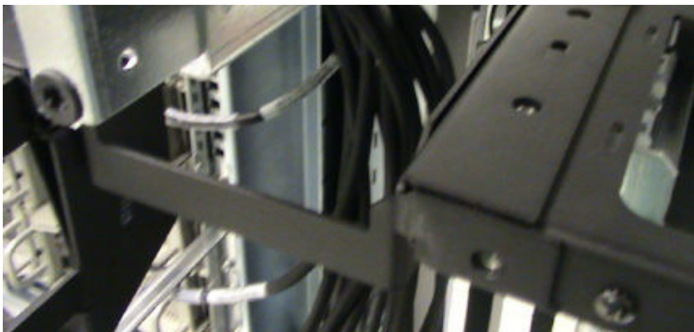
Figure 4-7 Rack Bonding Spacer – Top of Rack
